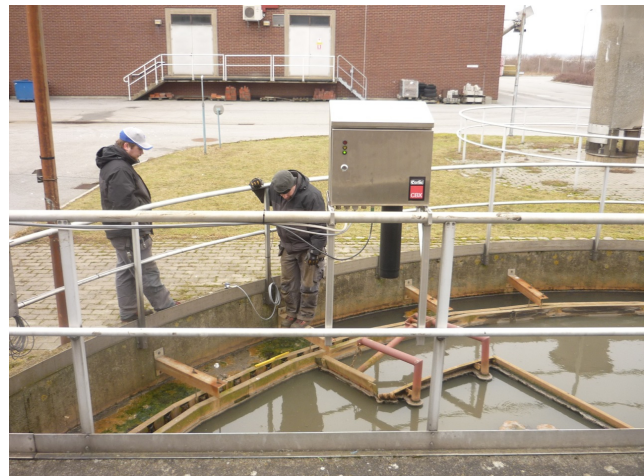
Outdoor installation at waste water treatment plant in Sweden
