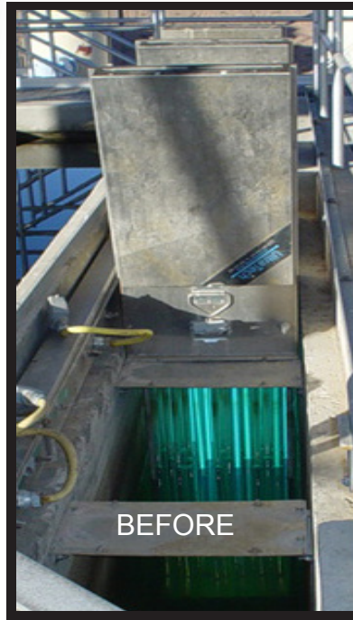
2003. Existing vertical plant using standard 65 watt lamps. Upgraded to high output 155 watt lamps. Allowed the plant to add automatic cleaning and to double flow.
