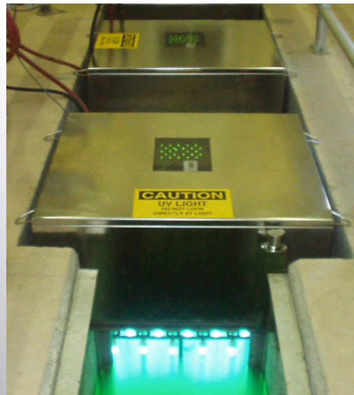
2003. Vertical plant using 65 watt lamps upgraded to amalgam lamps using 320 watts. This allowed the plant to meet more stringent discharge permit and increase their flows.
