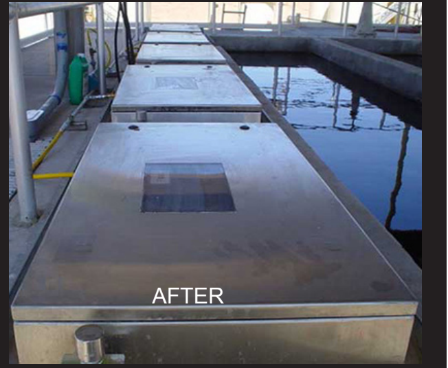
2003. Existing vertical plant using standard 65 watt lamps. Upgraded to high output 155 watt lamps. Allowed the plant to add automatic cleaning and to double flow.
