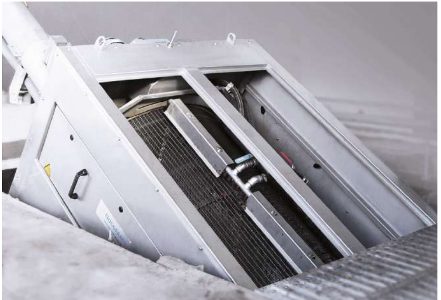
Rotary Drum Screen installed in channel
