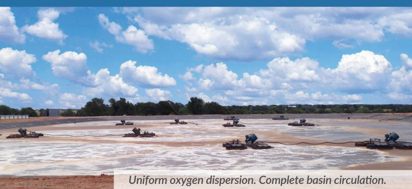
The Aire- $O_2^{\circ}$  Aspirator produces a horizontal and circular flow pattern, providing proven whole basin circulation. Improve your wastewater treatment with higher removal rates of Biochemical Oxygen Demand (BOD) and suspended solids.
