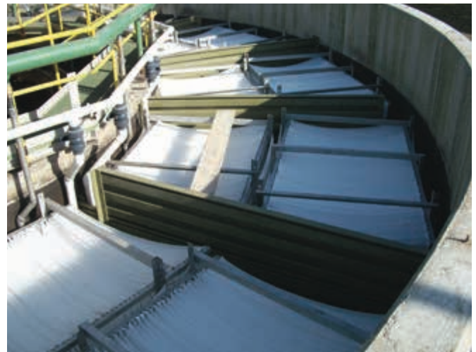
Treatment Stages with Fixed Biofilm Media
