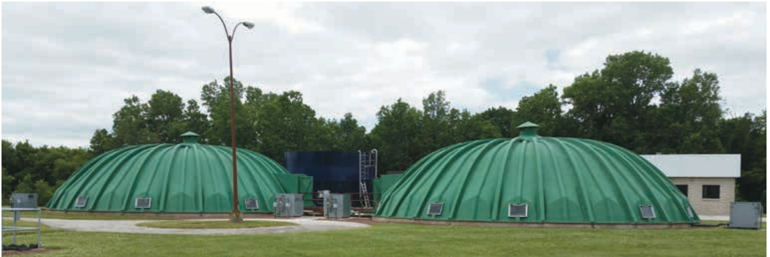
Northern Moraine Utility Commission, Wisconsin – Dome Covered Package Plants Retrofitted with Fixed Biofilm Media
