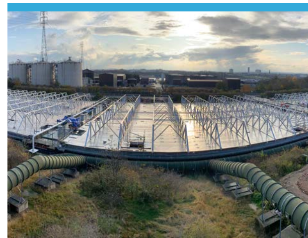
» Howdon Wastewater Treatment Works United Kingdom – Approximately 136,000 sq. ft.
