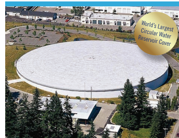
» Alderwood Water & Wastewater District Lynnwood, Washington – 375' Diameter
