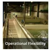
Gravity filtration allows for smooth flow with minimal disturbance of formed solids, which can be sheared through mechanical pumps and turbulent flow. Operators enjoy ease of access, whether for observation during treatment, or maintenance while out of service. Kurita America's Filtralator™ line of gravity filters provides a range of design possibilities with multiple options for underdrains, filter media and backwash type.
