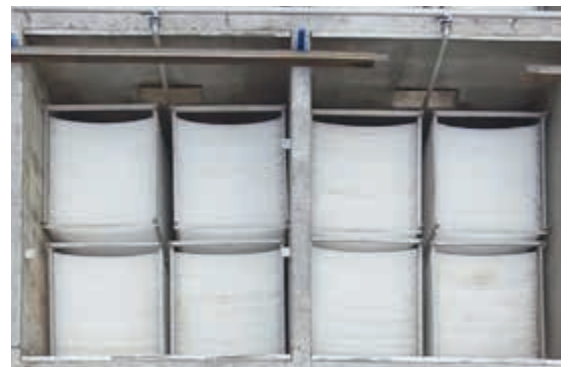
Nebula Biofilm Media Installation
