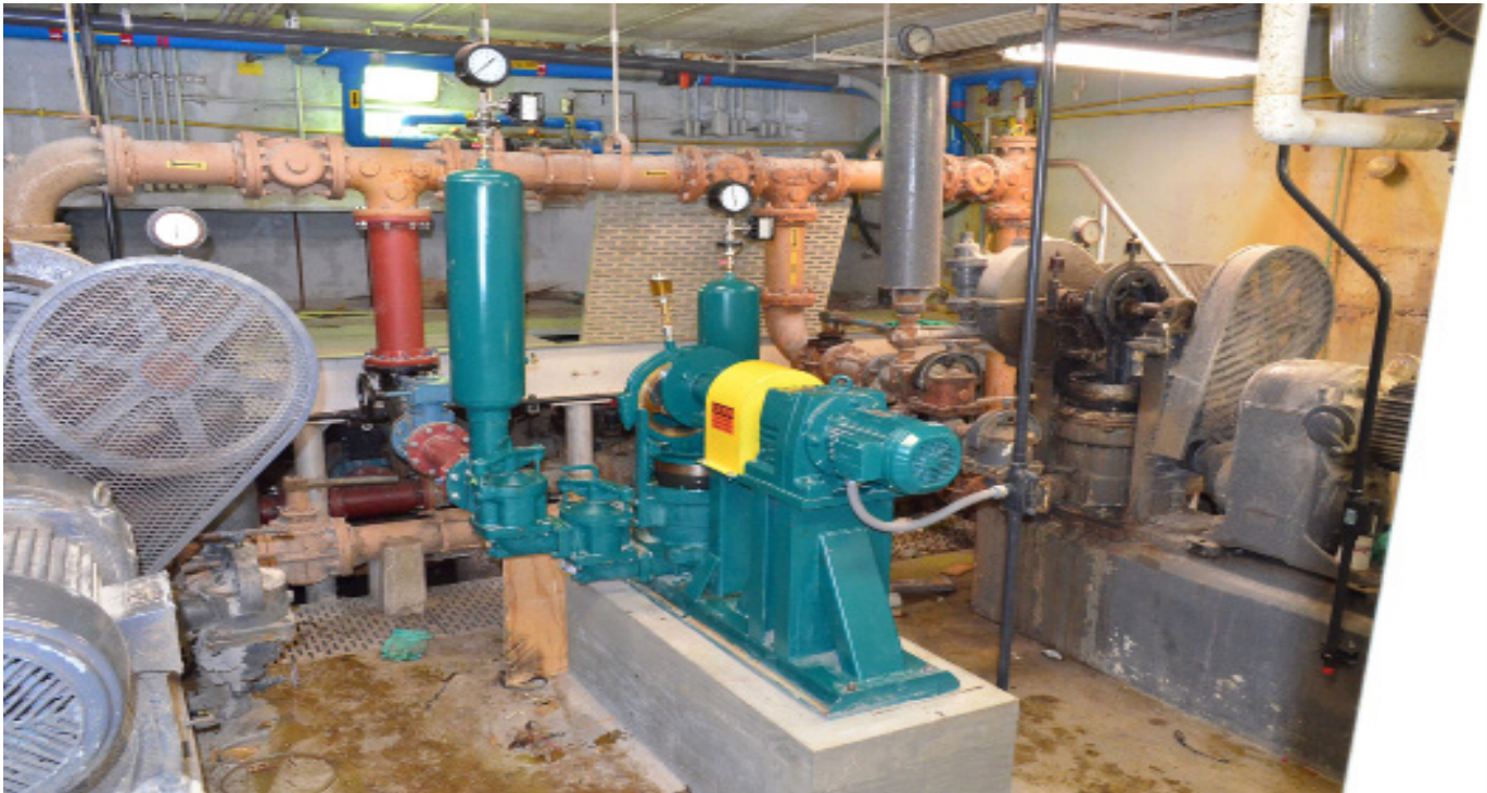
Model PE-941 dual ball valve at an upstate New York municipal sewage treatment facility. Facility upgrade involved upgrading control panels and pumping equipment. Wastecorp replaced Koline Sanderson and Carter plunger pumps. Dual ball valve configuration assists in pumping high solids above 15%.
