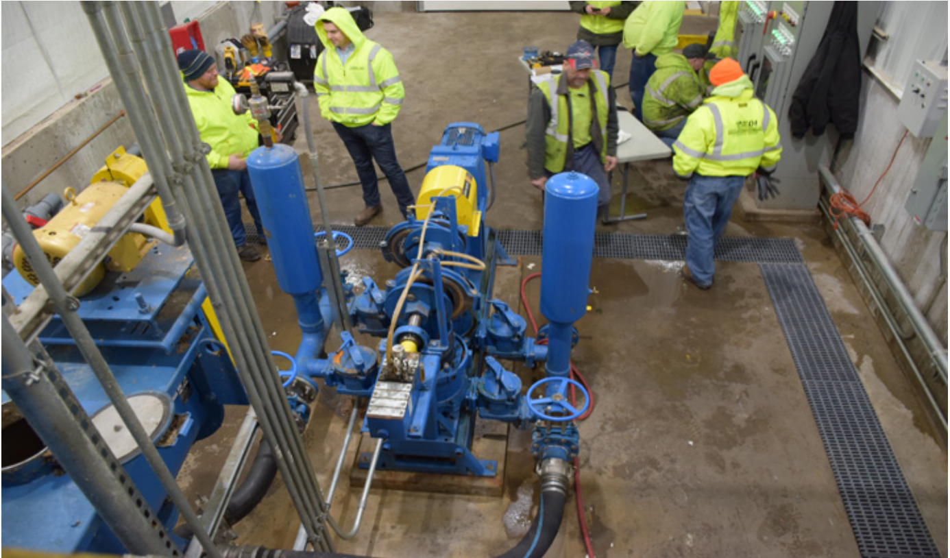
Wastecorp HPE 1142 plunger pump at an upstate New York sewage treatment facility. This facility has used plunger pumps for their primary sewage process for over 40 years. This new pump is a direct replacement.
