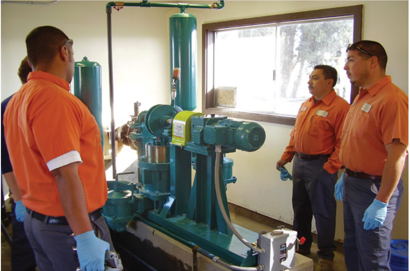
Wastecorp PE 941 plunger installation at a northern California wastewater treatment plant. Wastecorp offers start-up and staff training services from the factory or our worldwide dealer network.
