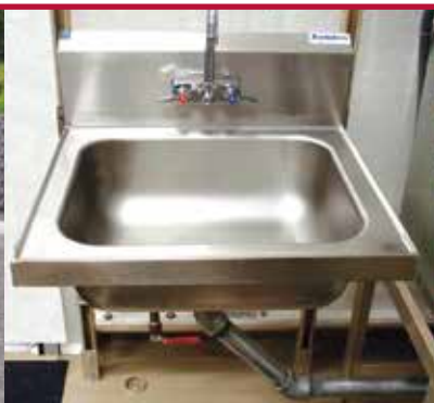
Water Basins / Drains
