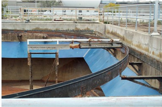
Density Current Baffles
