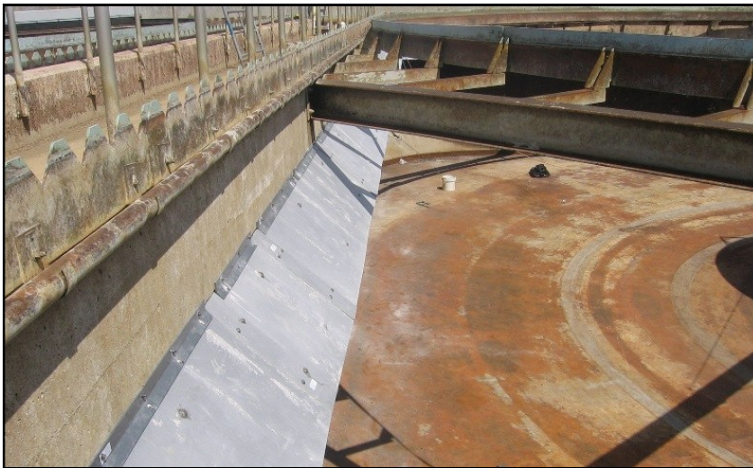
Density Current Baffles
