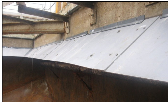
Density Current Baffles: Square tank installation
